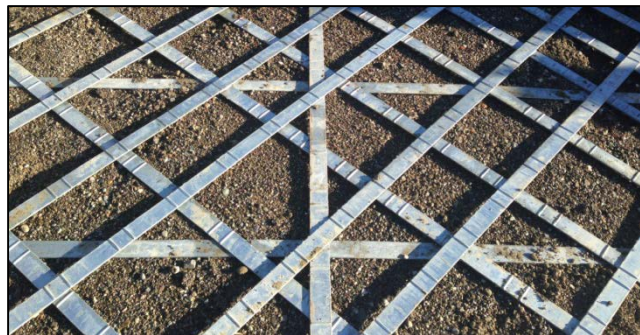
Fig. 5 Unusually high strip densities, angled and overlapped in corners.
