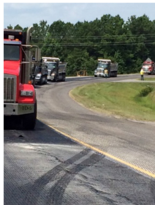
HaTelit® paving interlayers are durable allowing construction equipment to line up to the asphalt paving machine without "pick-up" under construction truck tires. Because HaTelit® interlayers are pre-impregnated, this aids in the asphalt tack rate application minimizing field construction issues.
