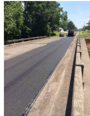
HaTelit® paving interlayers are made for full lane coverage. Here HaTelit® G50 was chosen in order to provide full lane width coverage allowing for uninterrupted paving operations to proceed without delay once installed.
