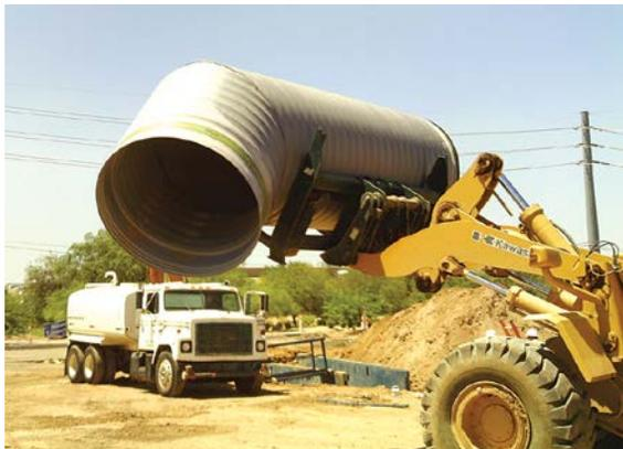
**A prefabricated section of ADS HP pipe is put in place for the road expansion project.**
