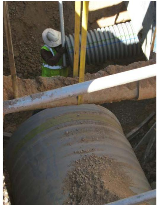
**The ability to easily install the ADS HP pipe enabled the crew to fit the new storm water drainage line under existing pipes. In one area, the 60-inch diameter corrugated pipe has been covered by 21 feet of fill.**
