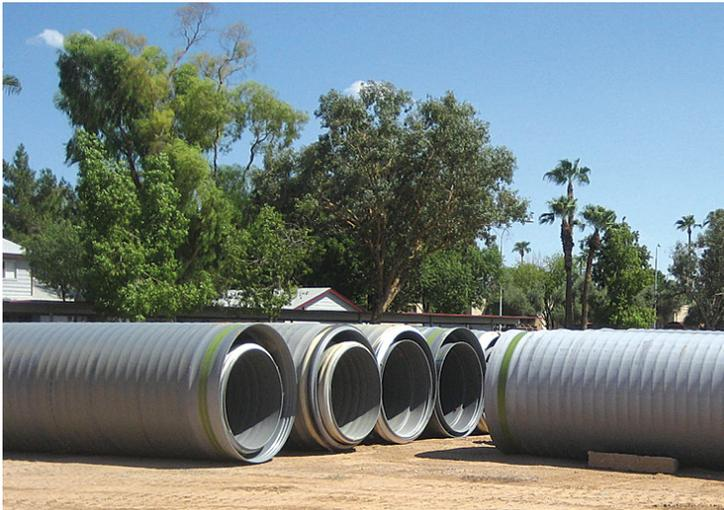
**For the deep burial of a road expansion's new storm water drainage line, highly-engineered corrugated pipe from Advanced Drainage Systems was used. The ADS HP pipe is designed and manufactured to handle heavy dead and AASHTO designated live loads. "Nesting" the different diameters of pipe reduced shipping costs and time.**
